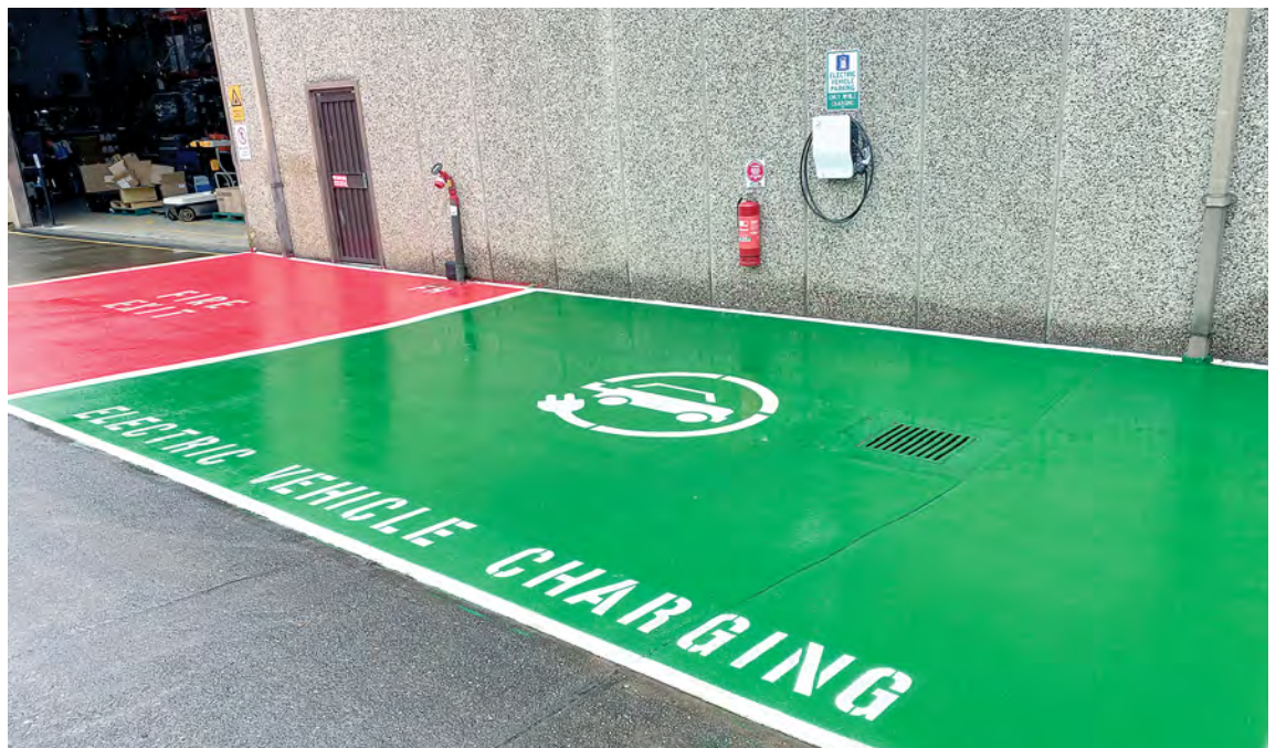
An EV charging station has been provided
