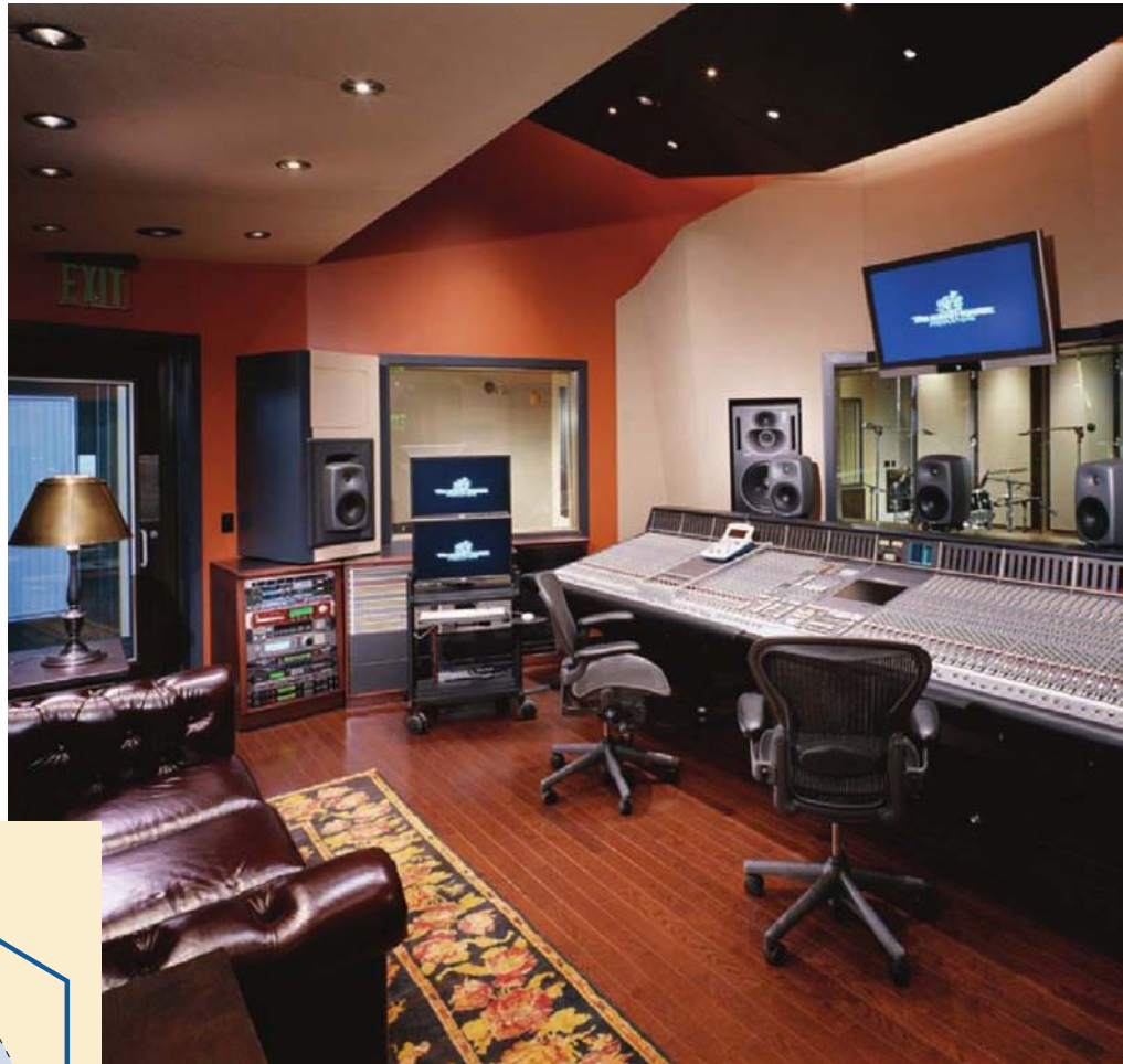
The multichannel audio control room shown here features flush-mounted stereo main monitors as well as a 5.1 surround system setup according to the ITU-R BS.775-1 standard. Note that the free-standing front left-center-right monitors are placed on separate stands to avoid vibration coupling between the console and the enclosures. The rear monitors are flush mounted in the side wall structure. Photo courtesy of WSDG Architecture and Acoustic Design.
