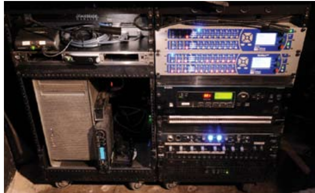
Four 14-space equipment racks can be rolled out from the enclosed area beneath the VIP section for maintenance, or moved to the FOH position for mixing.
